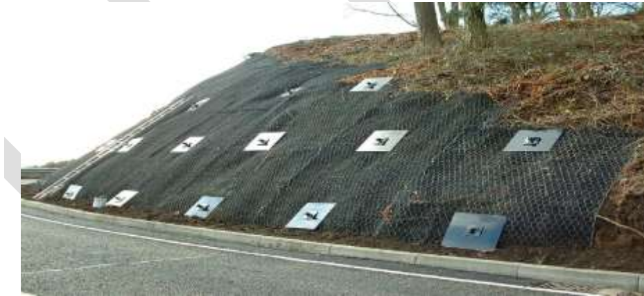
Figure 2: Actual picture of soil nailing in hill slope
