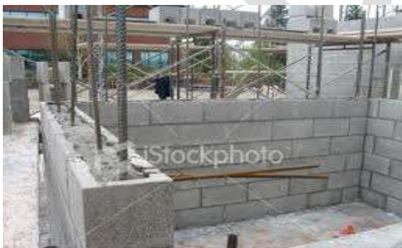
Fig 3: Concrete block walling
